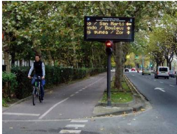
Picture 3: VMS panel in Paseo Bizkaia
