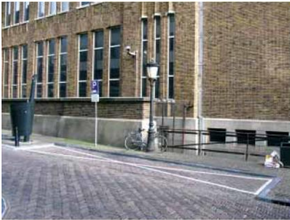
Figure 21: Cut-out in the footpath (sidewalk)/ in the roadway
