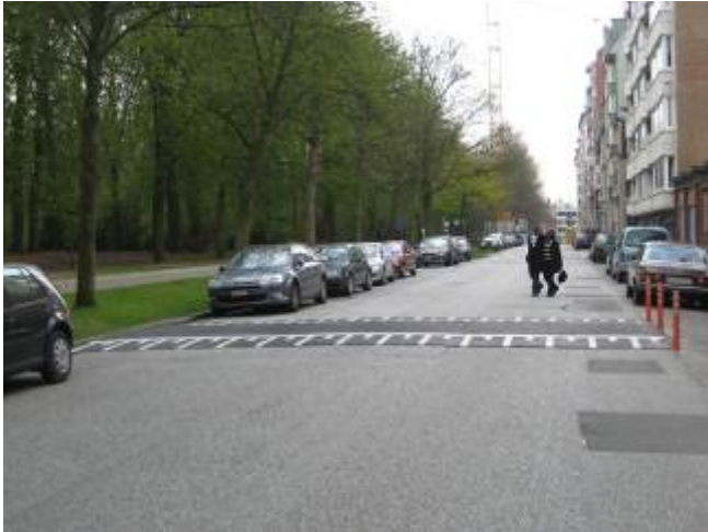
Picture 9: Leopold II-Laan: speed limiting measure
