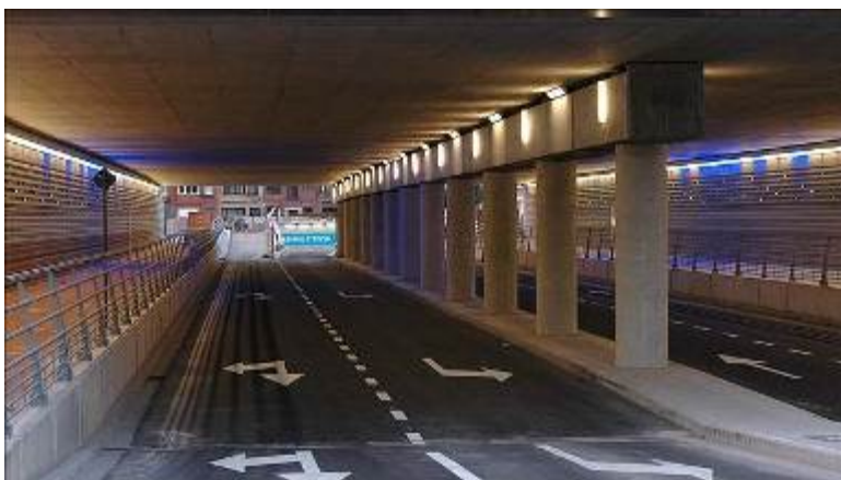
Picture 7: The new tunnel with the cycle lane (two directions) on the left side
