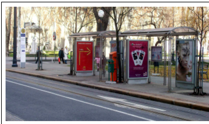
Typical PT station in Zagreb
