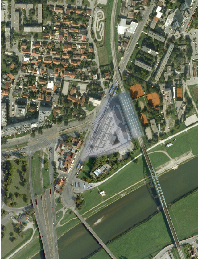
Aerial view of future Sava North Interchange
