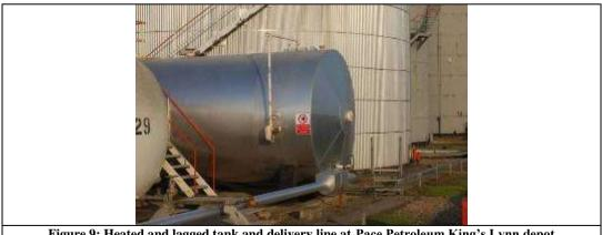
Figure 9: Heated and lagged tank and delivery line at Pace Petroleum King's Lynn depot
