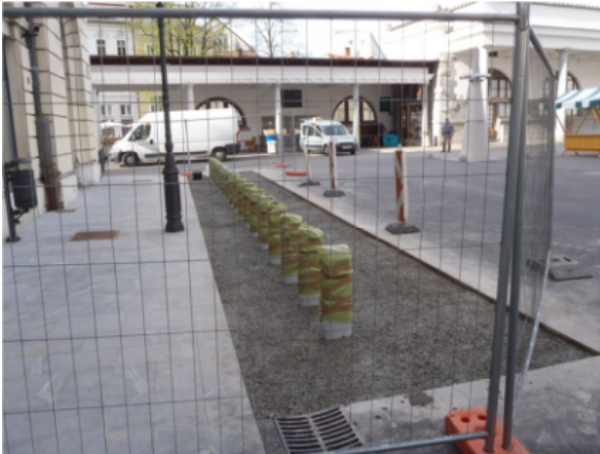
Image 1: City bike terminals in construction
