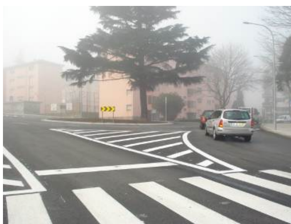
Picture 2: Roundabout on Dr. António Bernardino de Almeida street with Conde d'Avranches street intersection (after signalization)
