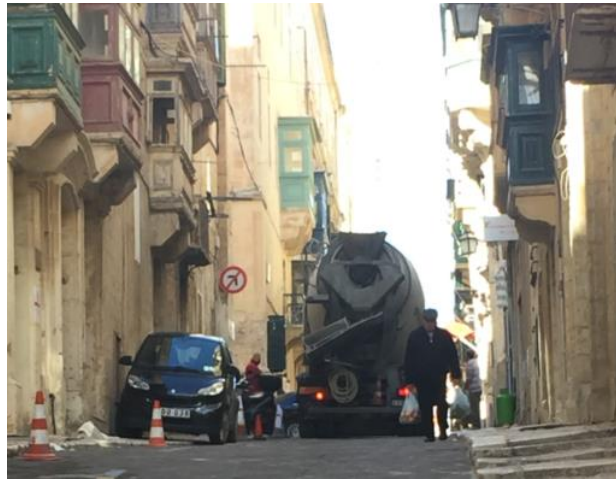
Figure 54: Use of large rigid truck for concrete delivery on construction site
