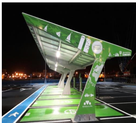
Figure 29: LPA 3.1 Charging Station
