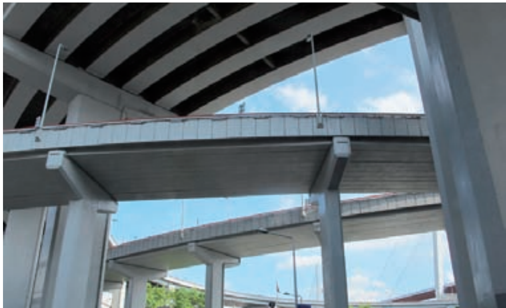
Road infrastructure in Shanghai
