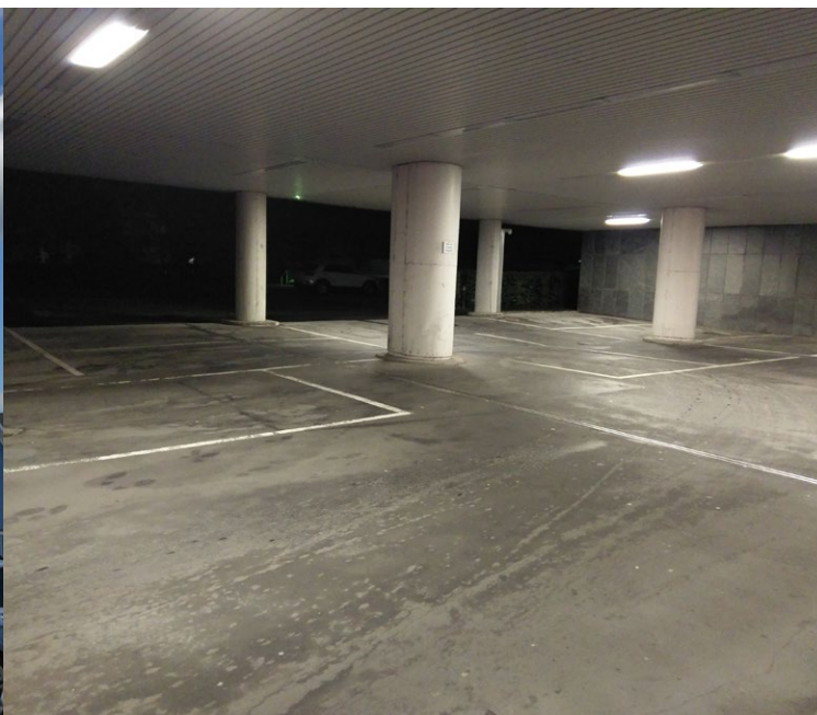
Figure 5: If on-street parking is free or cheap and readily available, nobody uses off-street parking. Source: Photo by Martina Hertel, Difu
