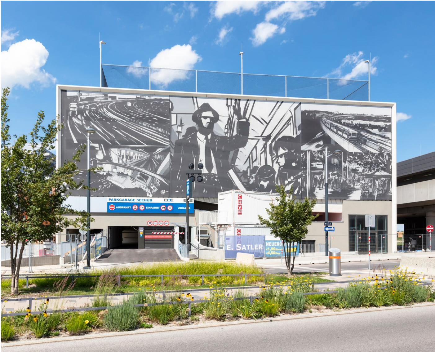
Figure 13: Shared Parking Garage in the Seestadt Aspern (City of Vienna, Austria). Source: © Daniel Hawelka
