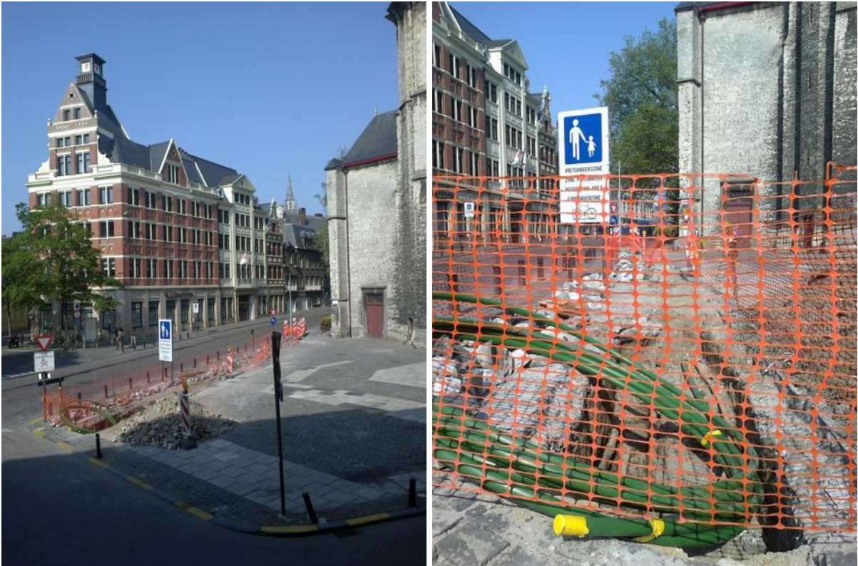
Photographs: Extension of the optical fibre network at St-Michielsplein
